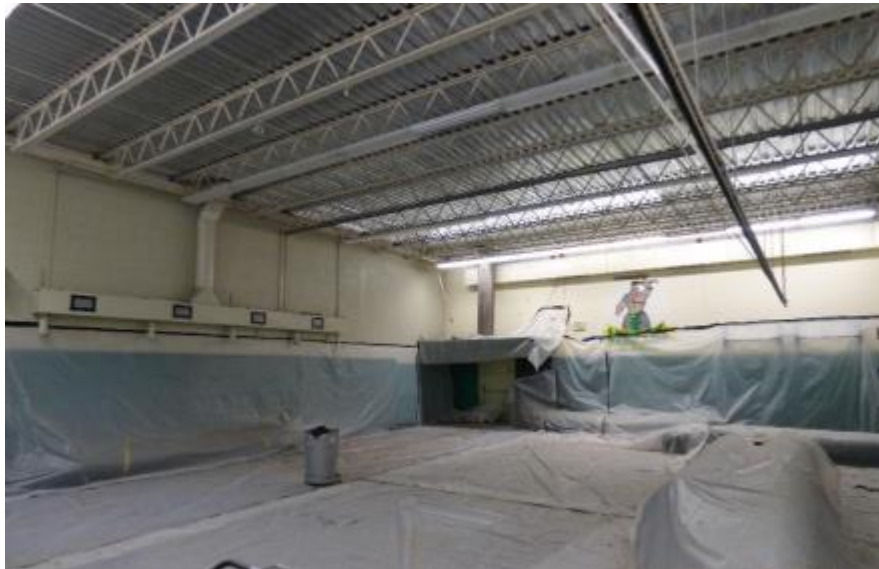
New Metal Roof Decking in Metal Shop
