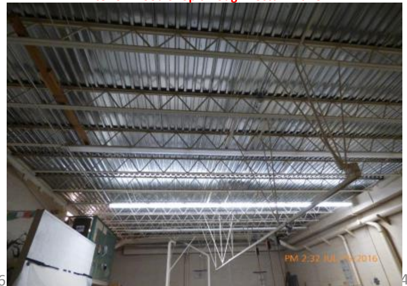
New Metal Roof Decking in Wood Shop
