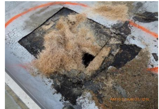
Cleveland HS - Deteriorated Tectum Decking Panel
