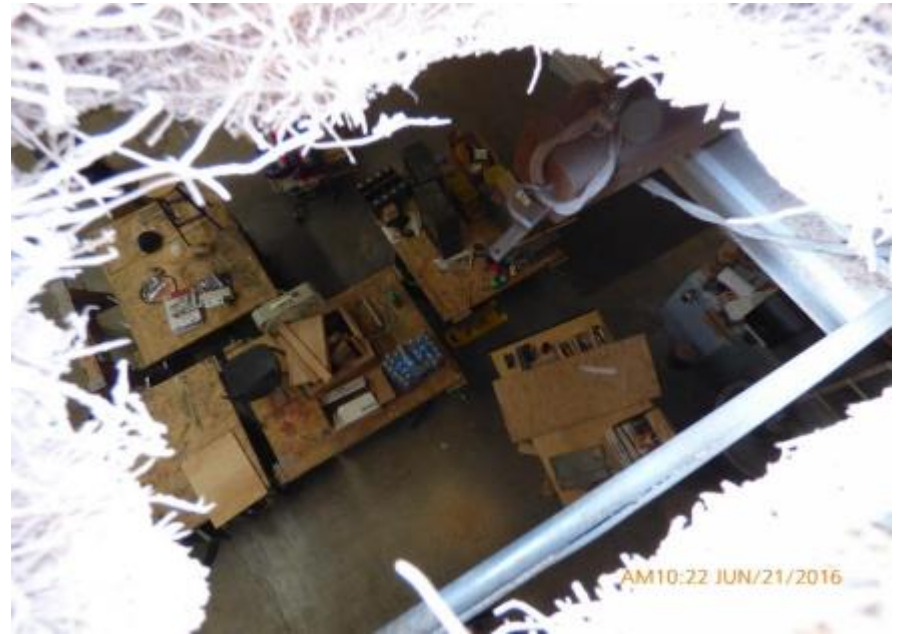
Interior Wood Shop through Tectum Panel
